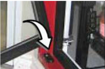
Figure 5 Insert Torque Rod
