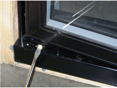
Figure 8 Release TorqueMaster Tension
