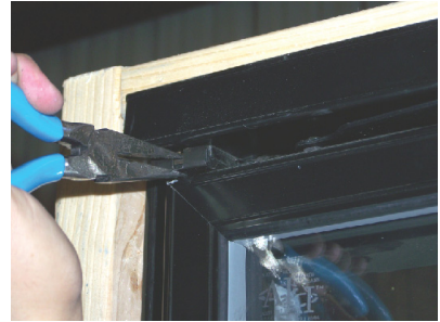
Figure 10 Disengage Hinge Pin
