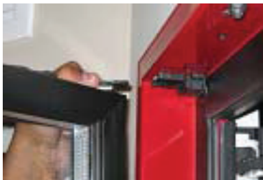
Figure 11 Withdraw Away From Hinge Gib
